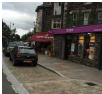
Attractive paved parking spaces, Windermere
